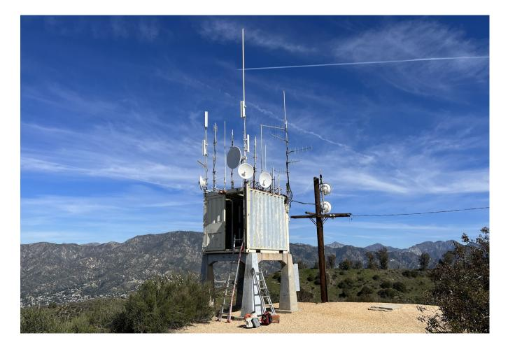
Large site (commercial) Pleasants Peak, California Yellow-highlighted gear is for mesh network. 360 degree user access, backbone links (not shown) + PTZ camera
