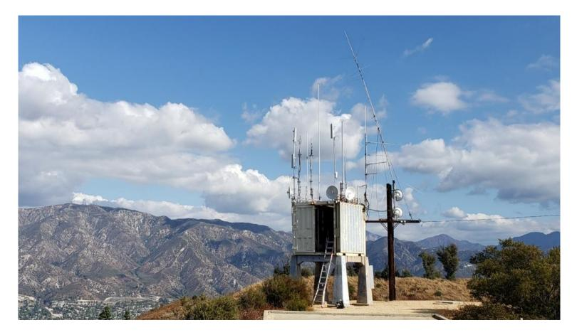
Large site (commercial) Pleasants Peak, California Yellow-highlighted gear is for mesh network. 360 degree user access, backbone links (not shown) + PTZ camera
